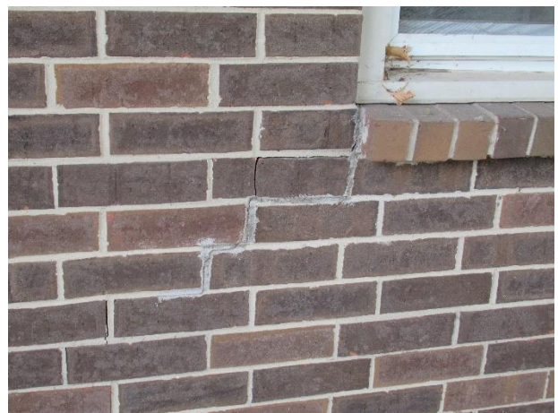
Masonry and mortar step cracks, note previous repairs
