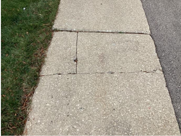
Sidewalk cracks near clubhouse
