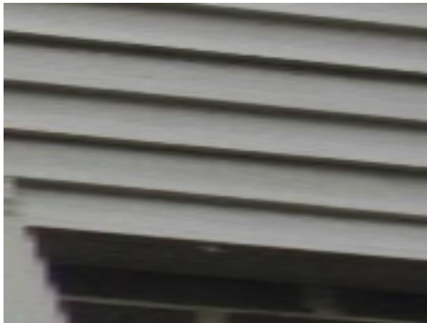
Weathered and deteriorated wood components
