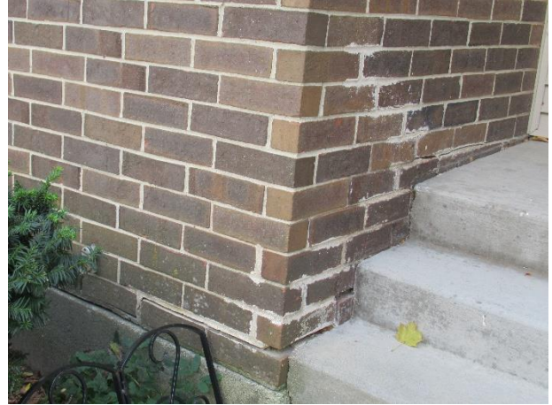
Previous repairs, separation of mortar and masonry, and stoop settlement. Unit 212 shown.
