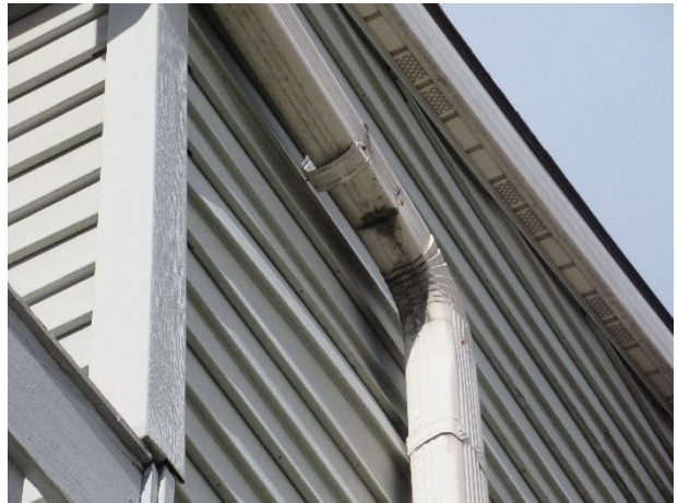
Evidence of leakage at seams
