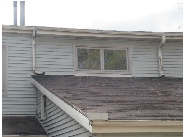
Three-tab shingles, note weathering and granular loss
