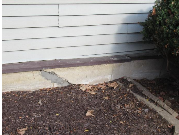
Previous foundation repair
