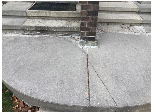
Sidewalk cracks Units 106 - 108
