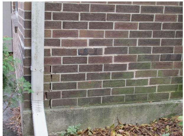
Mortar and masonry step cracks and previous repairs
