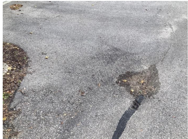
Isolated pavement deterioration
