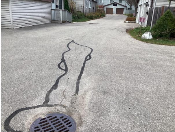
Pavement overview, note centerline drainage cracks and previous repairs
