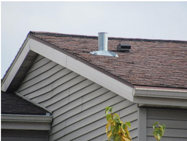
Shingle lift and weathered shingles
