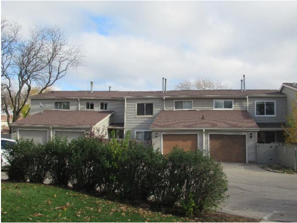
Asphalt shingle roof overview, note deflection in roofs likely due to building settlement
