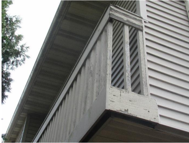
Weathered and deteriorated wood components
