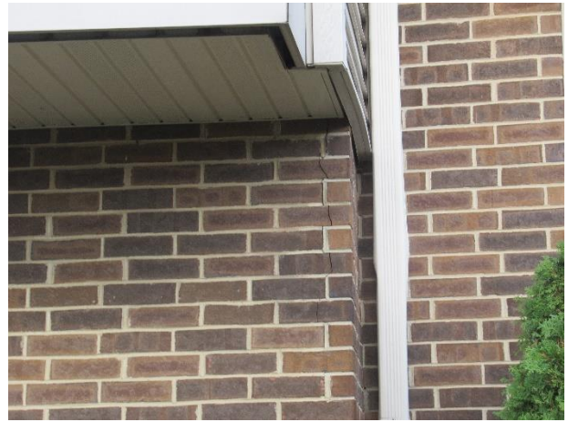
Vertical cracks, Unit 246 shown
