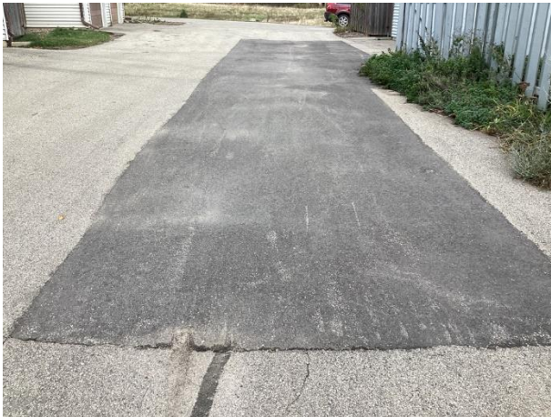
Isolated significant patch
