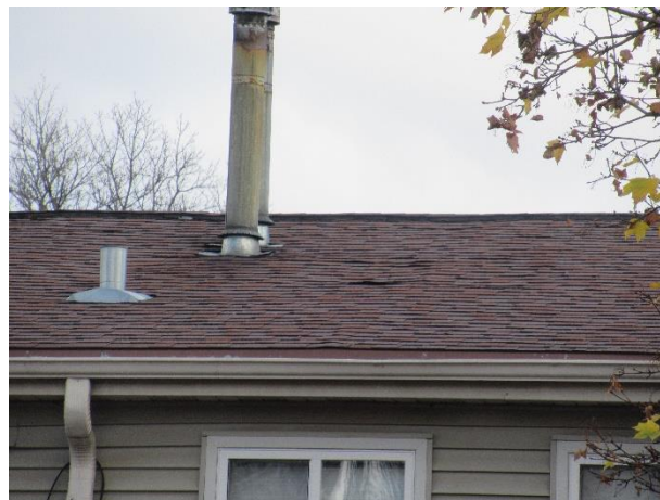
Shingle lift and weathered shingles
