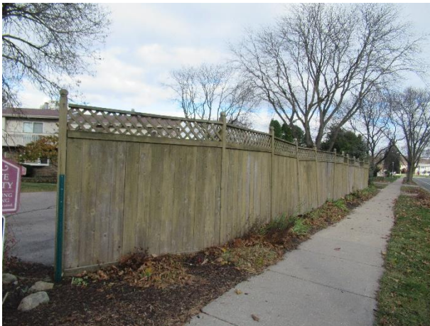
Grand Canyon Drive fence, note deflection and faded finishes
