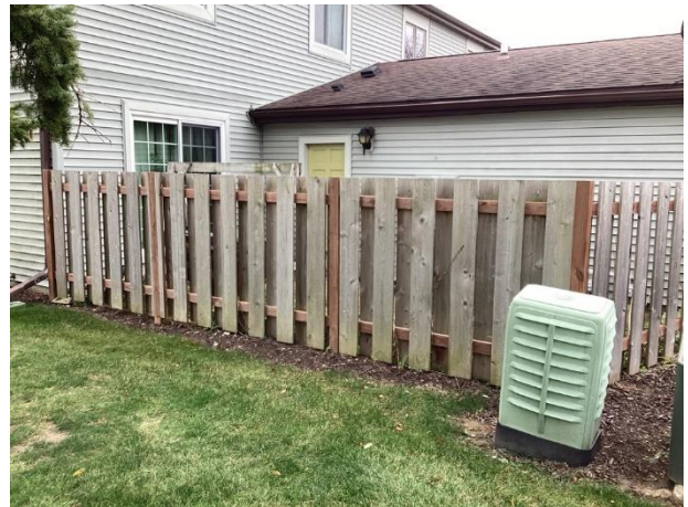
Replaced wood fence posts at patio
