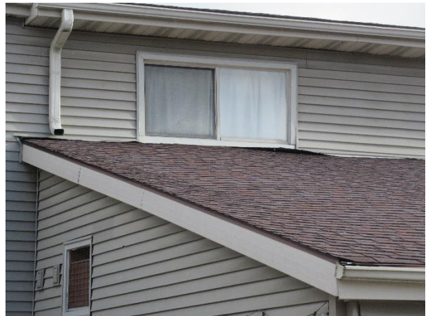
Lifted flashing detail
