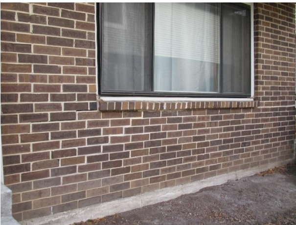
Masonry bowing and mortar bed separation at Unit 212
