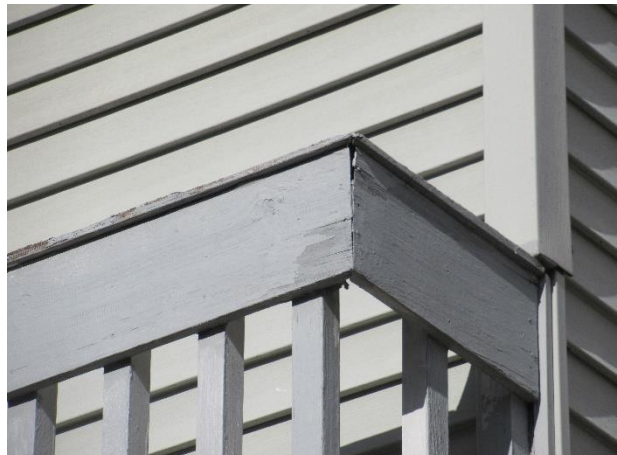
Weathered and deteriorated wood components
