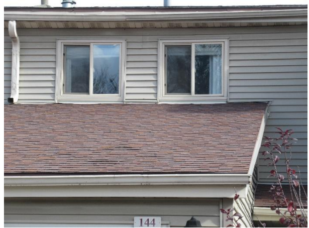
Shingle lift and weathered shingles
