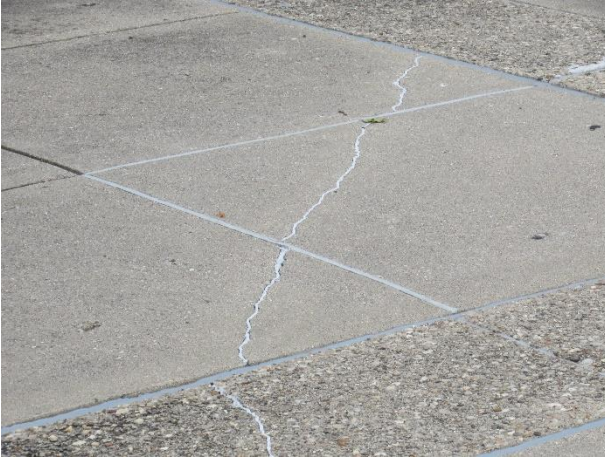
Previous cracks repairs
