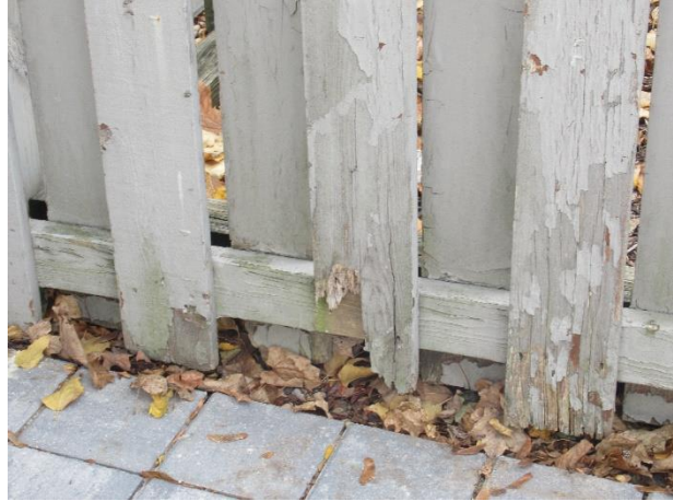
Fence deterioration
