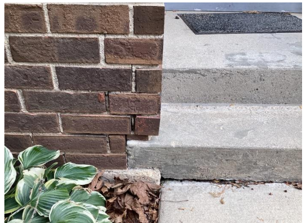
Mortar deterioration and missing mortar at Unit 214
