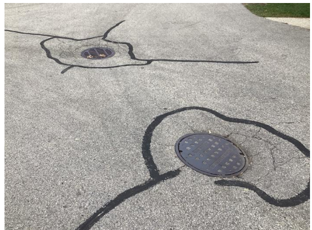
Minor catch basin settlement, note pavement cracks
