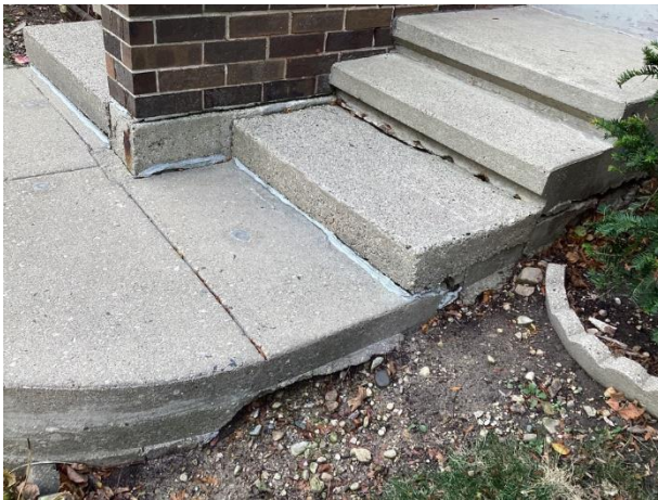
Soil undermining at Unit 112 sidewalk
