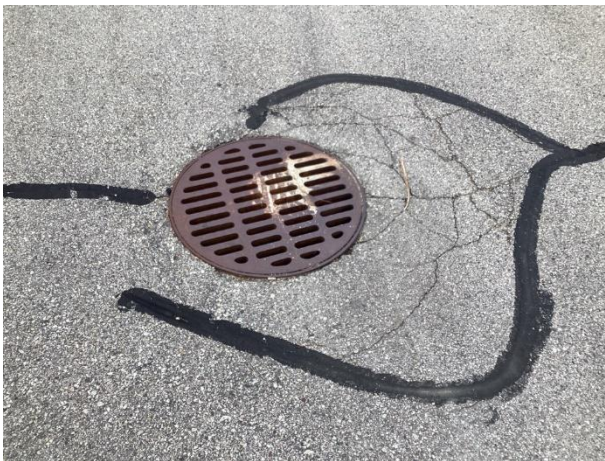
Catch basin settlement, note pavement cracks
