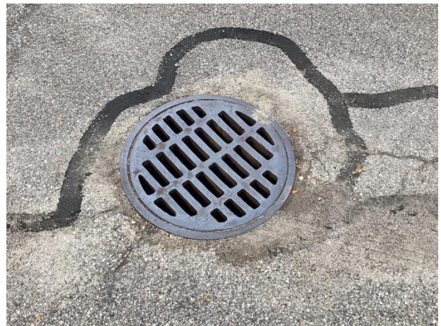
Catch basin settlement, note pavement deterioration
