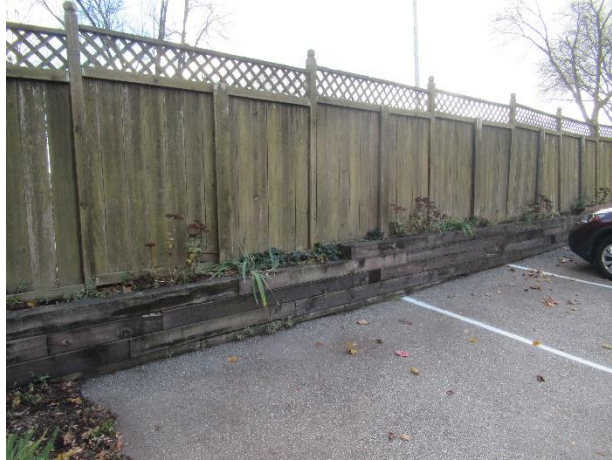
Timber retaining wall
