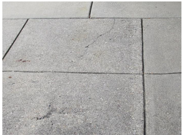
Deck cracks
