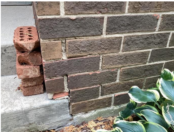
Mortar deterioration at Unit 214
