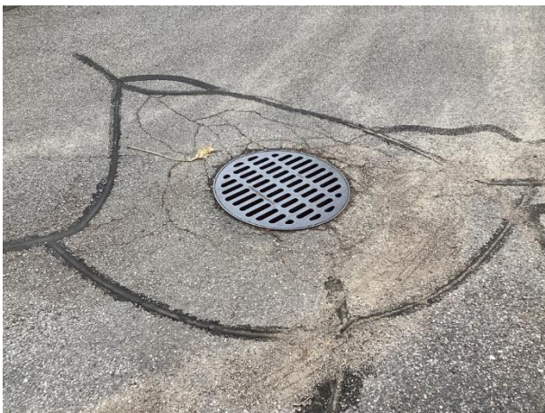
Catch basin settlement, note pavement cracks
