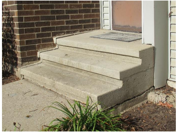
Significant stoop settlement, note cracks along wall and slab, Unit 226 shown
