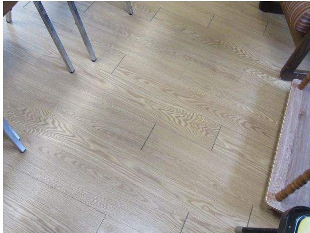
Gaps at seams (photo from 2020 inspection)
