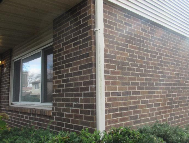
Step cracks at two elevations, Unit 216 shown
