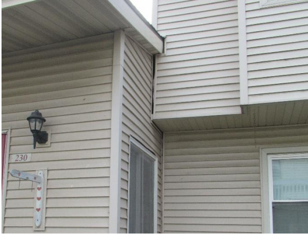
Gaps, note separation between Units 230 and 232
