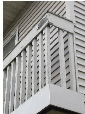
Peeling finishes and wood deterioration
