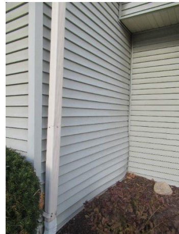
Warped/bulging siding, Unit 224 shown
