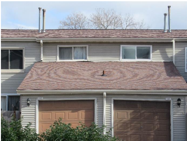
Roof (building) deflection, note lifted flashing and downspout discharge onto shingles
