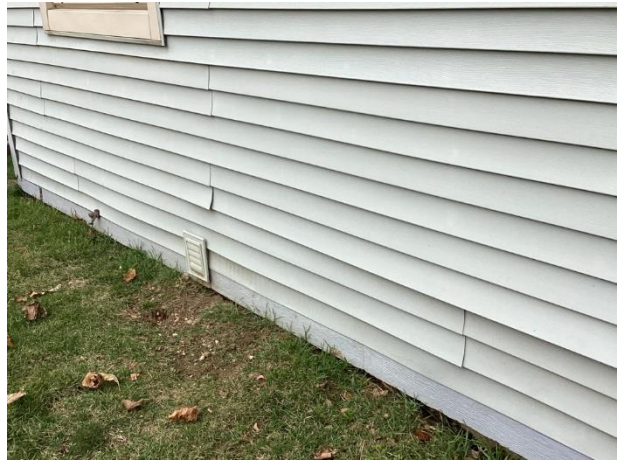
Siding lift at Unit 214
