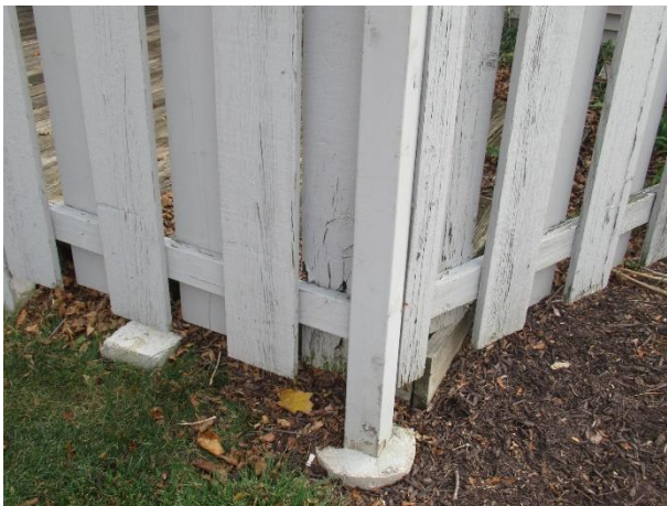
Fence wood deterioration
