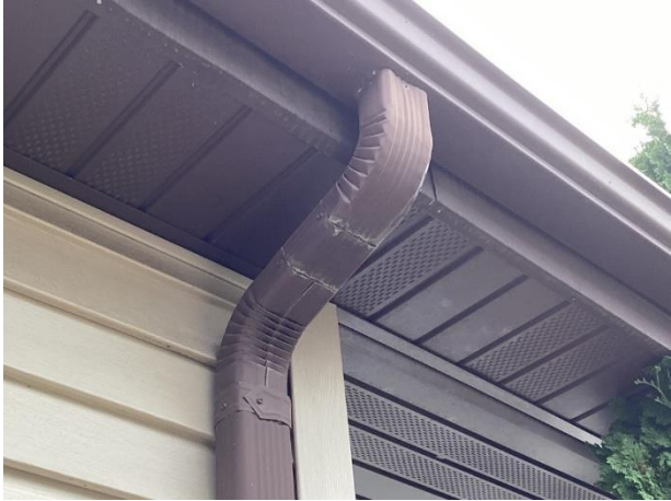
Evidence of leakage at seams at clubhouse
