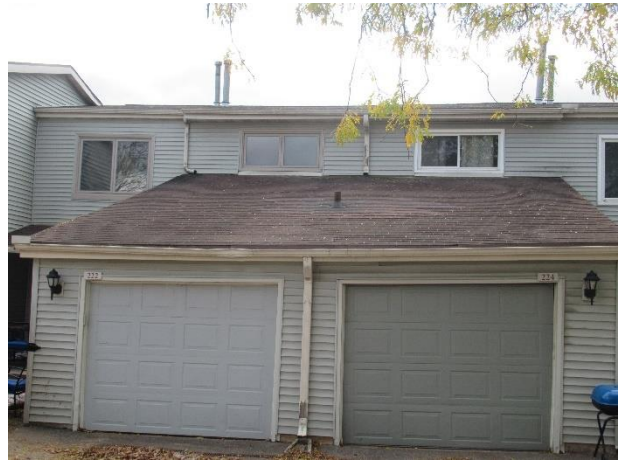
Weathered shingles, repairs and apparent garage settlement
