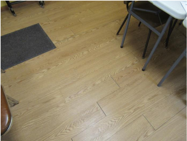
Gaps at seams (photo from 2020 inspection)
