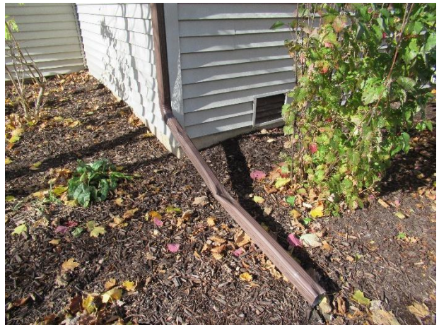
Damaged downspout
