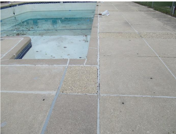
Pool deck overview, note sealant deterioration
