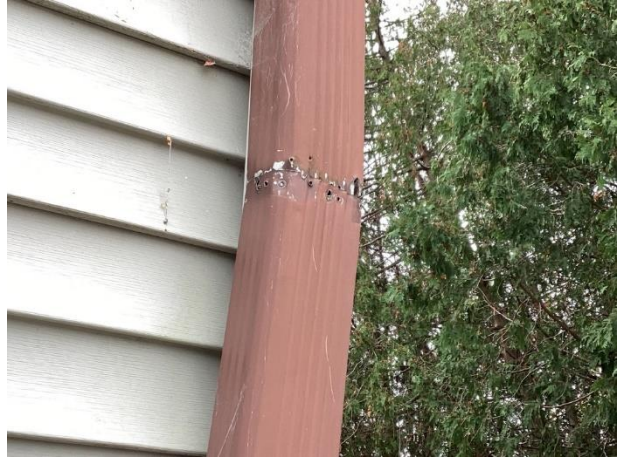
Multiple fastener holes
